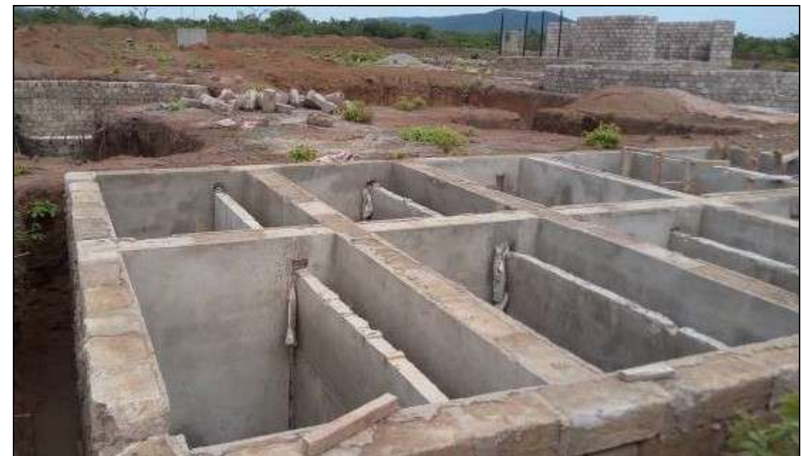
Plate 7.3: Liquid waste disposal system under construction in Geita Town
